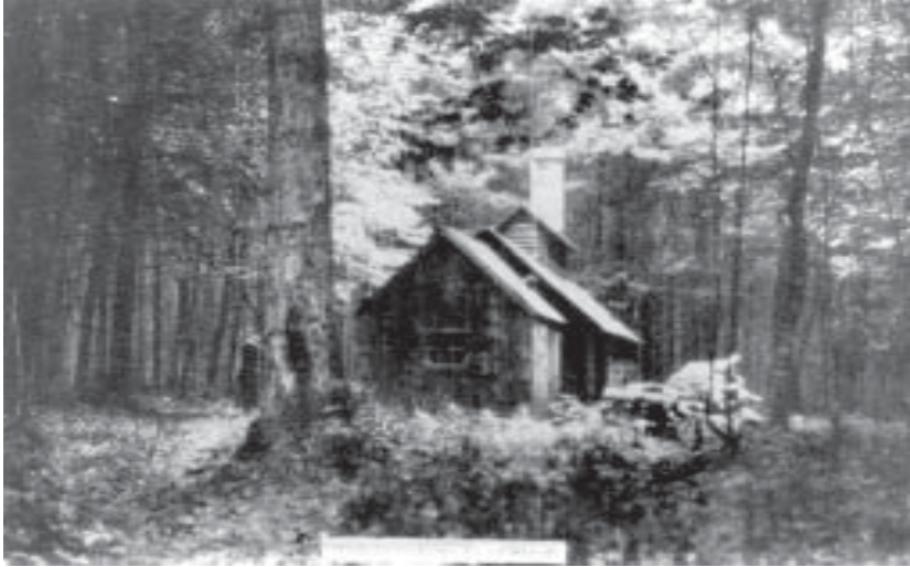
FIGURE 4. Undated real photo postcard of sugarhouse at Camp 1, note the larger cupola, tall rectangular smoke stack, and absence of sap unloading ramp (Uncataloged Postcard. Photo used with permission of the John M. Longyear Research Library of the Marquette County Historical Society).
